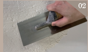
02 平批一遍，控制在一个颗粒厚度，表面均匀 半干后收光至表面平整 Batch once, control to ensure uniform particle thickness After semi drying, let it shine until the surface is smooth
