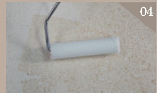
04 罩面层(推荐使用极致哑光罩面)，均匀 辊涂两遍（加水10-15%） Cover layer (recommended to use ultimate matte cover) uniform Roll coating twice (add 10-15% water)
